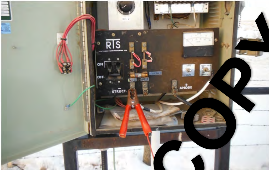
2-23 Direct hook-up to a structure cable (positive feeder cable)
