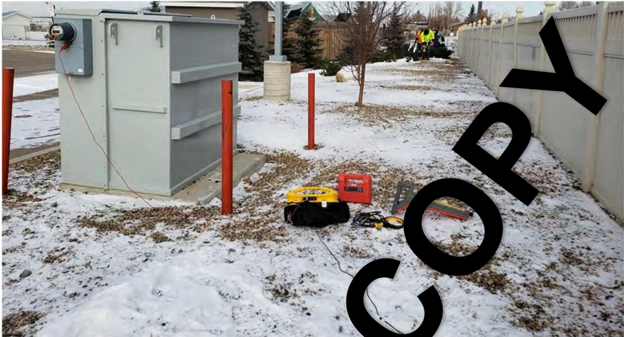
2-19 Direct connection to the meter at a transformer
